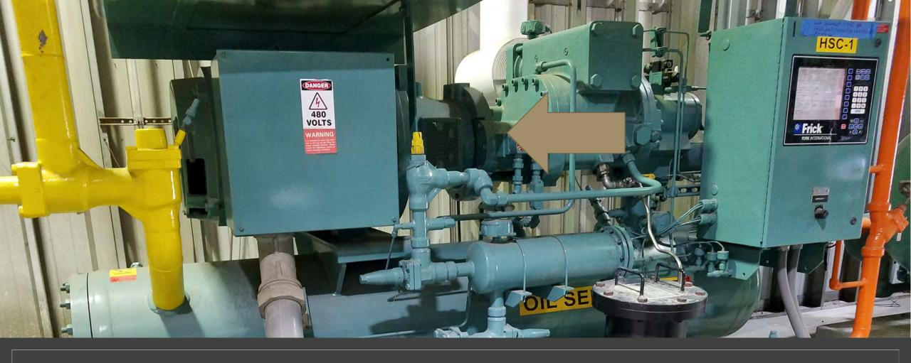
Inspect for rotor axial play in motor driven rotor shaft (annual)
