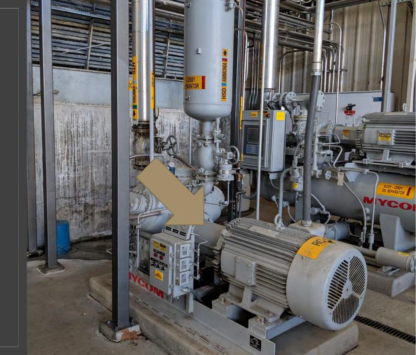
Visually inspect starter connections and associated timers and relays
