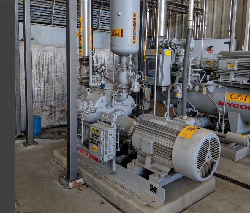
Measure (hot) compressor-motor drive shaft alignment (annual)
