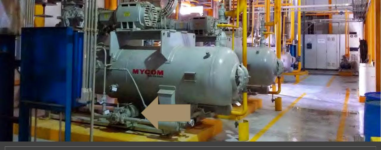
Lubricate compressor and external oil pump electric motor bearings (semi-annual)
