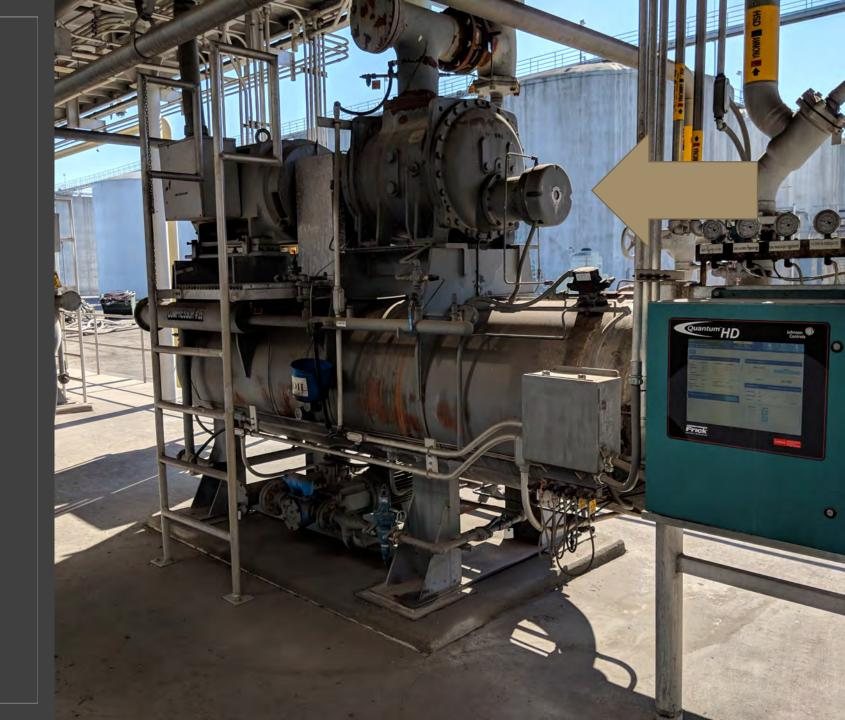
Inspect alignment of motor drive shaft
