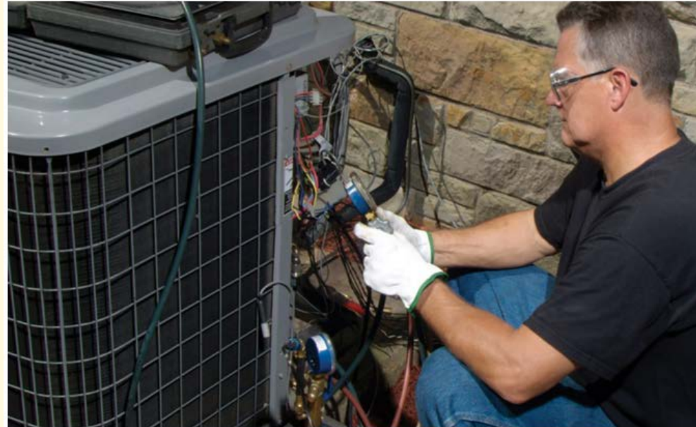
REFRIGERANT RETROFIT: An HVAC technician retrofits a residential air conditioning unit from R-22 to Freon™ MO99. Photo courtesy of the Chemours Co.
